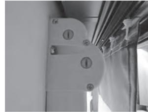
Do not leave the blinds closed over a longer period of time. Should a blind lose its tension over a period of time, use a flat screwdriver to retighten the tension spring on the blind. Insert the screwdriver and turn it clockwise one or two revolutions.
